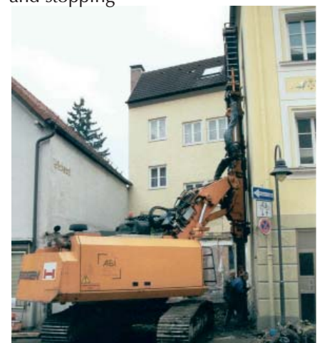
ABI resonance-free vibrator right against an adjacent structure
